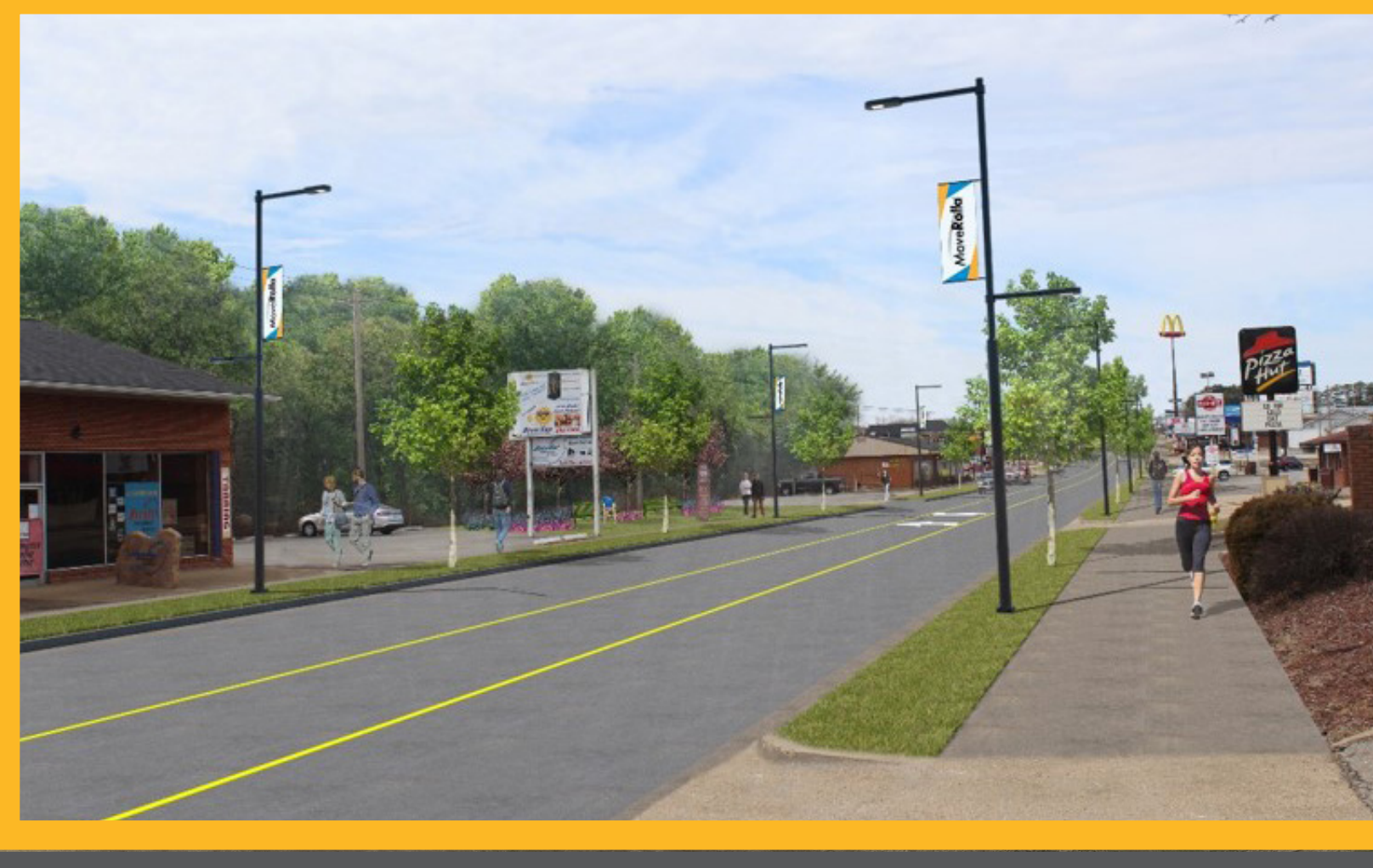
Utilities and Aesthetics: Power lines will be removed along the corridor. New lighting and a 8-foot bike and hike trail on the north side of the corridor will be constructed and a 5-foot sidewalk on the south side.
